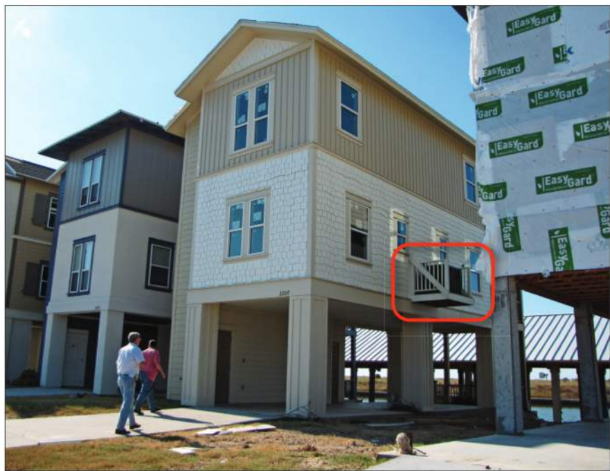
Figure 4-3. Elevated HVAC condenser unit on cantilevered platform (Port Bolivar, Texas).
