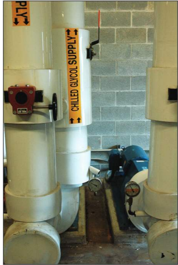
Figure 5-4. Chilled water pump, Georgetown, Delaware.
