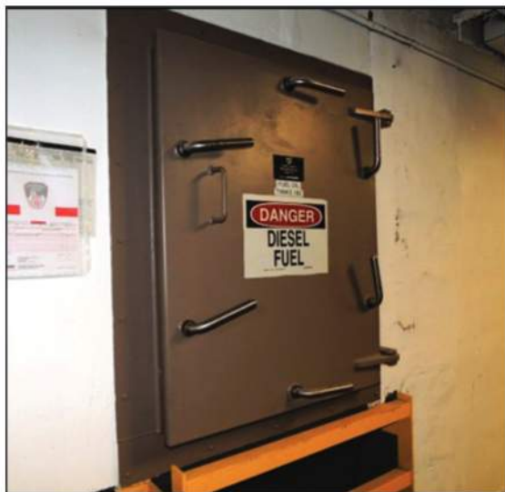
Figure 5-23. Fuel tank placed in floodproof vault in basement of commercial high-rise (New York, NY).
