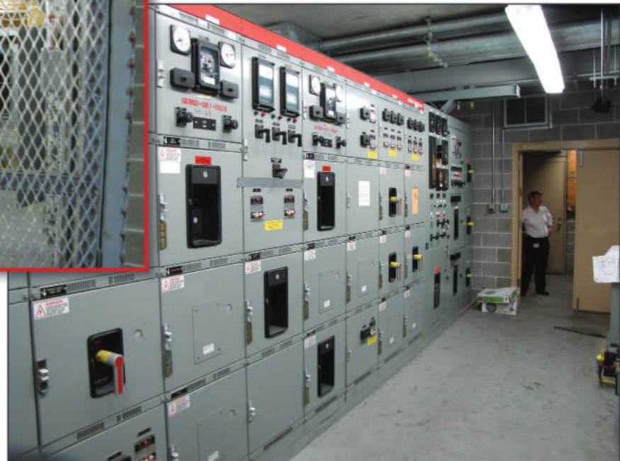
Figure 5-15. Exterior view (top left) and interior views (bottom right) of elevated emergency generator and switchgear at medical center in Galveston, TX. Figure 5-14 is an exterior view of the electric room.
