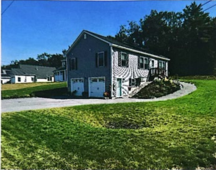
Photograph 9 – Unknown Drainage Structure in Front of 15 Kapok Street (Photo Taken by Jaime Wallace, PE Dated September 26, 2023)
