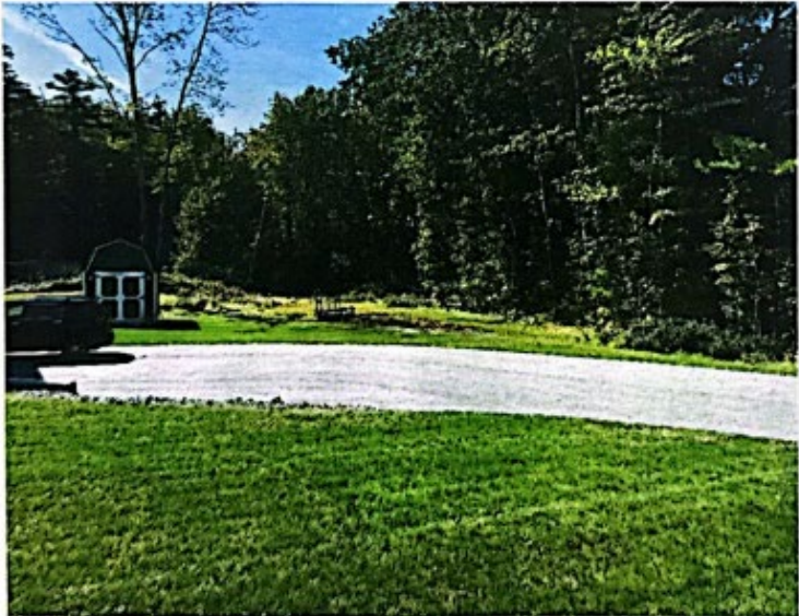
Photograph 4 – Location of Proposed Maintenance Access Road to Wet Pond (Photo Taken by Jaime Wallace, PE Dated September 26, 2023)
