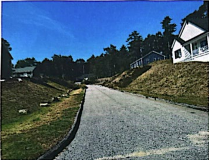
Photograph 13 – Juniper Street Looking West (Photo Taken by Jaime Wallace, PE Dated September 26, 2023)
