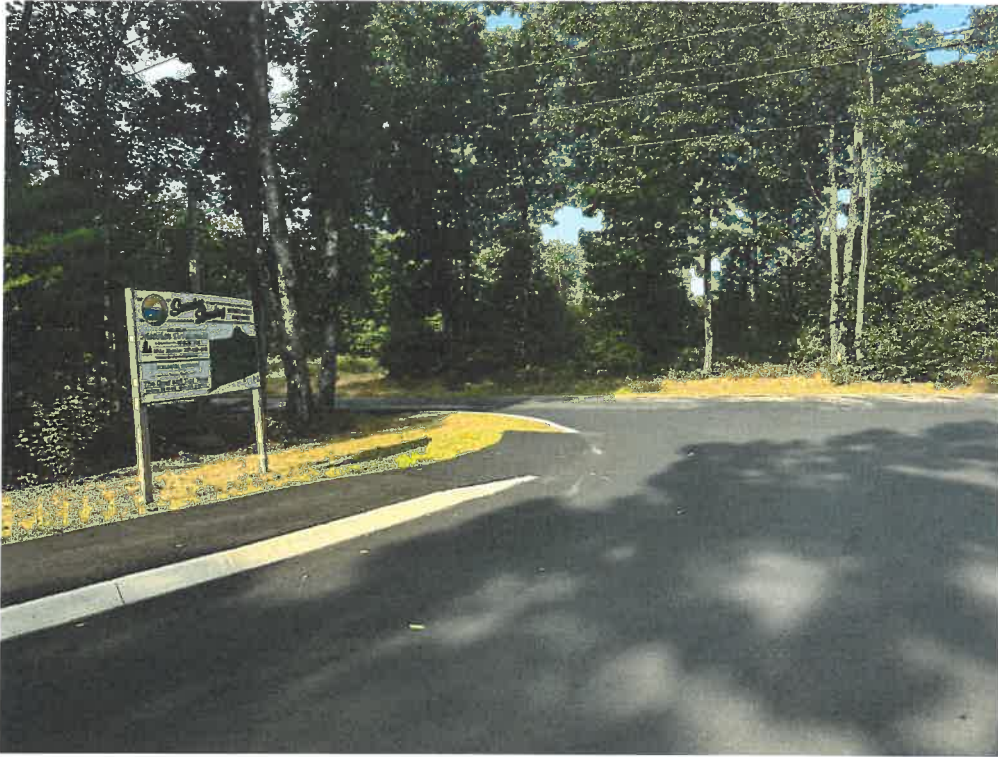
Photo 1: Handicap Detectable Device Needed at Intersection of Summer Long Drive and Ross Road (Photo taken by Jaime Wallace, PE dated 9/13/2024).
