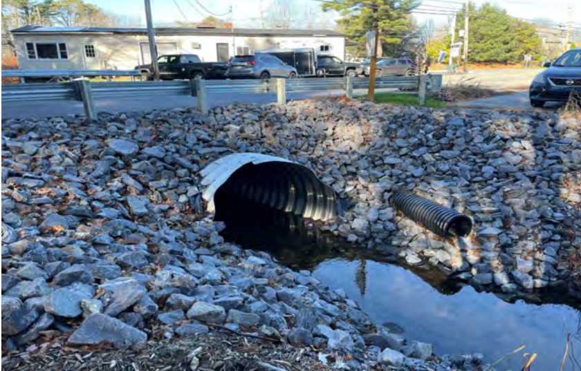
Photo of the culvert during construction.
