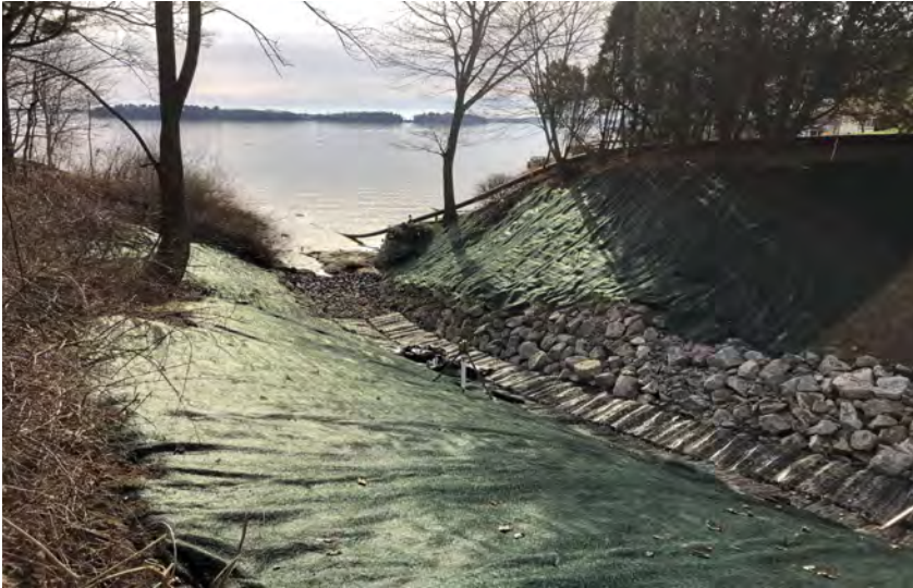
Improvements to Underwood Road Drainage Outfall
