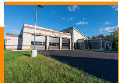
LEWISTON FIRE SUBSTATION Lewiston, ME
